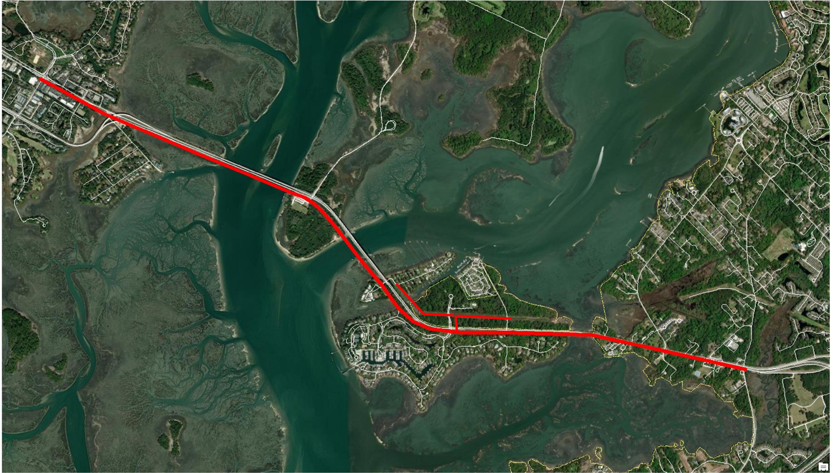
3-lane roadway from Moss Creek to Spanish Wells – lifeline bridge (3-lanes with accommodations for 4th lane)
