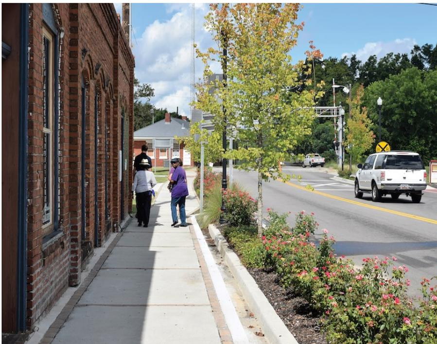
**Sidewalks:** The primary purpose of sidewalks is to provide a safe path for pedestrians that is separated from vehicular traffic by on-street parking or a planting strip. Width of sidewalks should be a minimum of 5 feet in low density residential areas and increase in width in areas of high pedestrian traffic. Sidewalks should be prioritized where they provide safe and convenient access for pedestrians to schools, parks, retail, and services.
