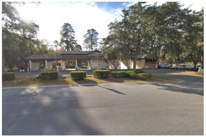
Figure 2: Existing Condition of Site from Drive Aisle
