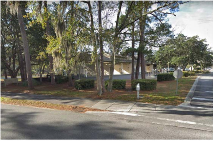
Figure 1: Existing Condition of Site from Office Park Road
