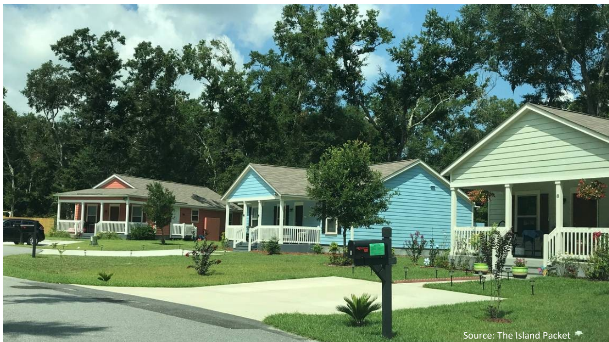
Figure 2. Phase 1 of The Glen neighborhood constructed by Habitat for Humanity, Hilton Head Island, SC
