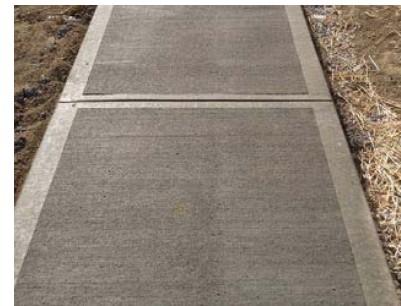
Concrete Walks- Tooled w/ Broom Finish
