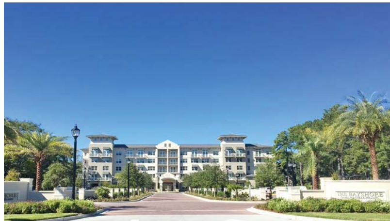
Entry Road to align with Phase 1
