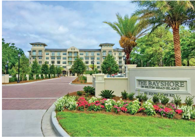
Stucco Entry Walls and Signs to match Phase 1
