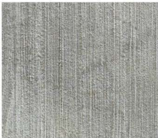
Concrete Sidewalk With Broom Finish
