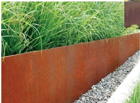
Steel Retaining Wall With Mow Edge
