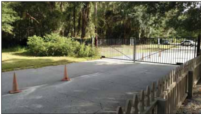
VIEW FROM ZIPLINE TICKETING OFFICE TOWARDS EXISTING PARKING LOT
