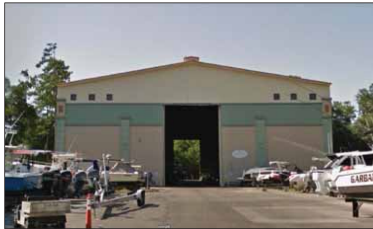
BROAD CREEK MARINA - BOATHOUSE STORAGE BUILDING
