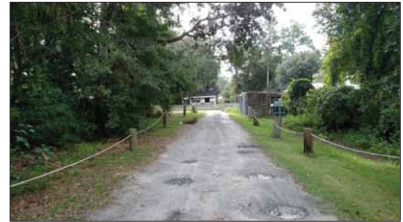
VIEW DOWN EXISTING GRAVEL DRIVE TOWARDS EXISTING TICKETING BUILDING
