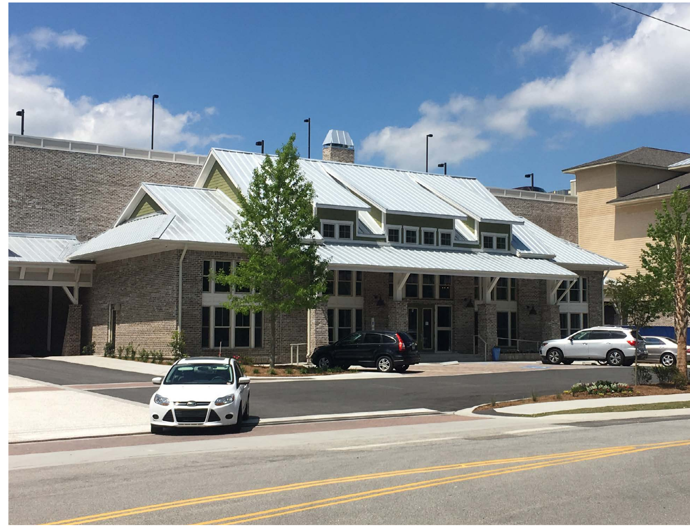
LOWCOUNTRY DORMERS / CLUBHOUSE ROOFLINE
