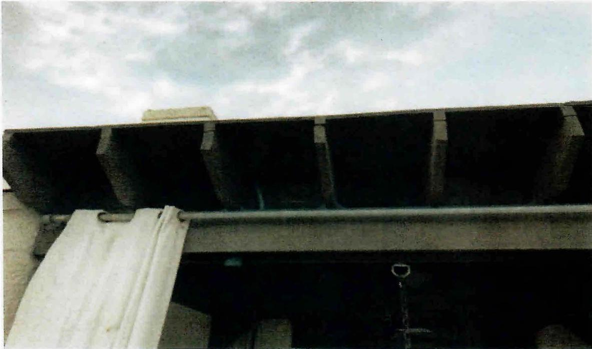
This is the side of the canopy facing Palmetto Bay. Blocks are to be placed between the ceiling rafters, on top of the beam at every space between the rafters and nailed as shown in the previous detail. This is to be done with all ceiling rafters.
