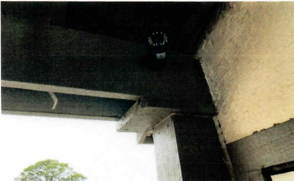
This is typical of the westerly outside post and beam connection. On both ends of this beam, the beam must be tied to the post with 16-gauge coil strapping, that is 12 inches long on each member (post and beam). The post is to be anchored to the wall with HDG  $\frac{1}{2}$ " carriage bolts. A block is to be placed on the sheetrock wall on the inside to span between not less than 2 existing wall studs. 1" HDG washers are to be used on the bolt. Place 3 bolts @ 18" o.c. in the wooden post.
