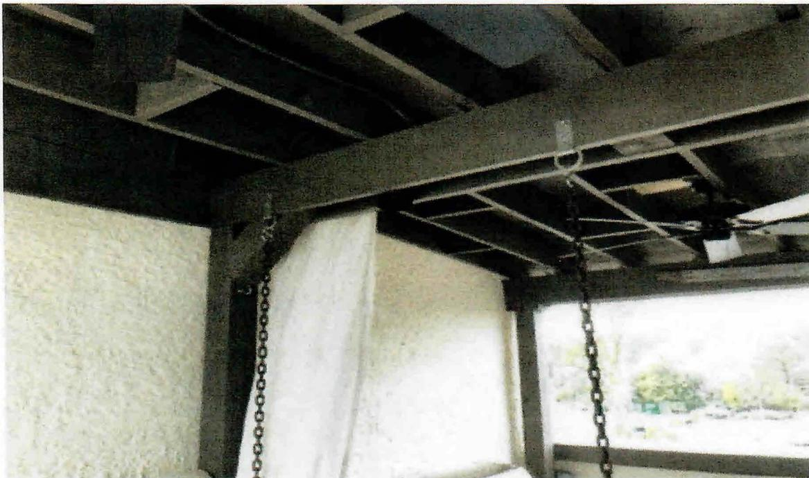
The post to the right in the picture above is closest to the exterior of the deck and it too, needs to be bolted to the concrete block wall with  $\frac{1}{2}$ " red head bolts with a minimum penetration into the block wall of 5". The red head is to be epoxied into place with Simpson 2-part epoxy or equal. Place 3 bolts @ 18" o.c. in the wood post.
