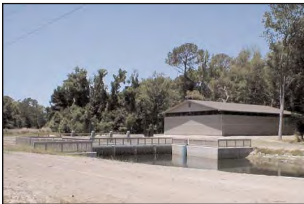
FIGURE 3-14: JARVIS PUMP STATION
