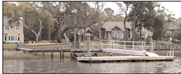
FIGURE 5-2: TYPICAL OLDER DOCK
