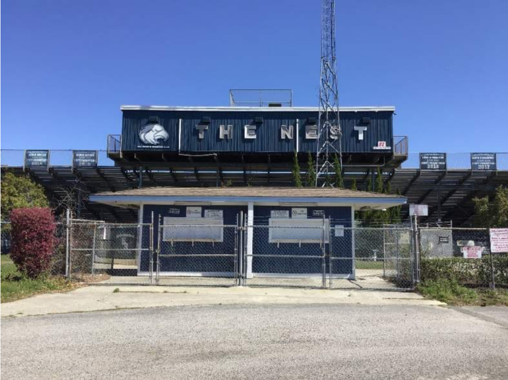
Existing Football Press box and Ticket Booth
