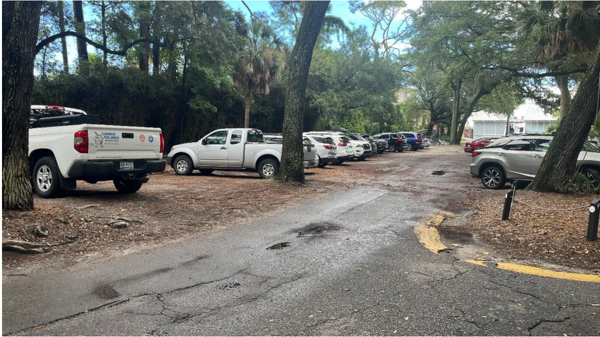
Existing Parking Lot
