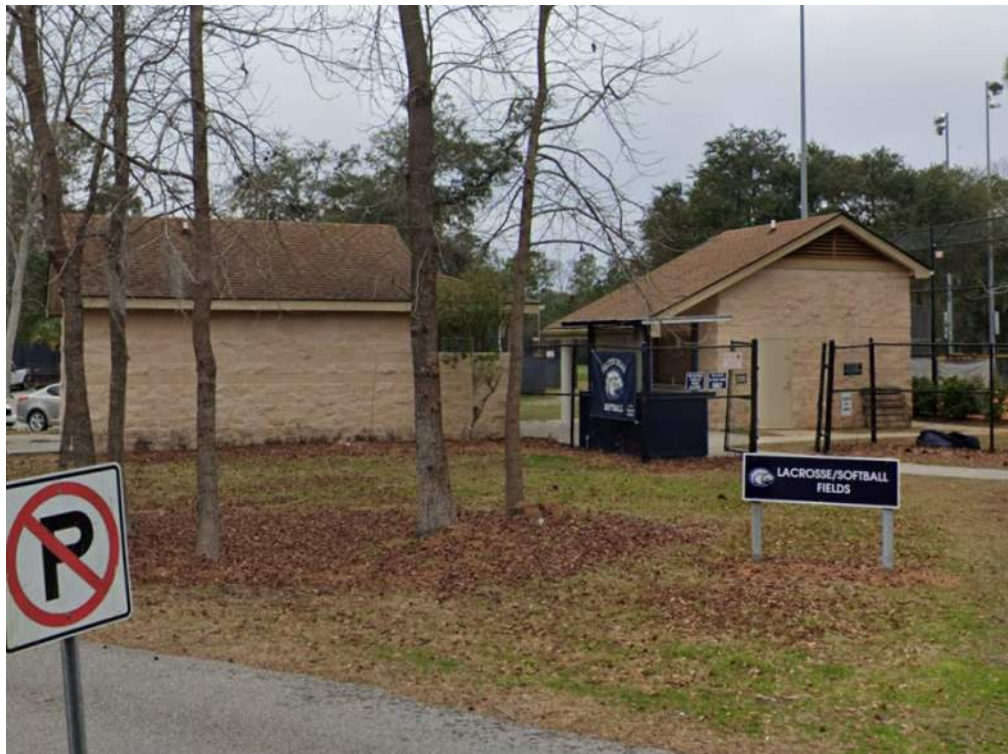
Existing Softball Pressbox and Toilets
