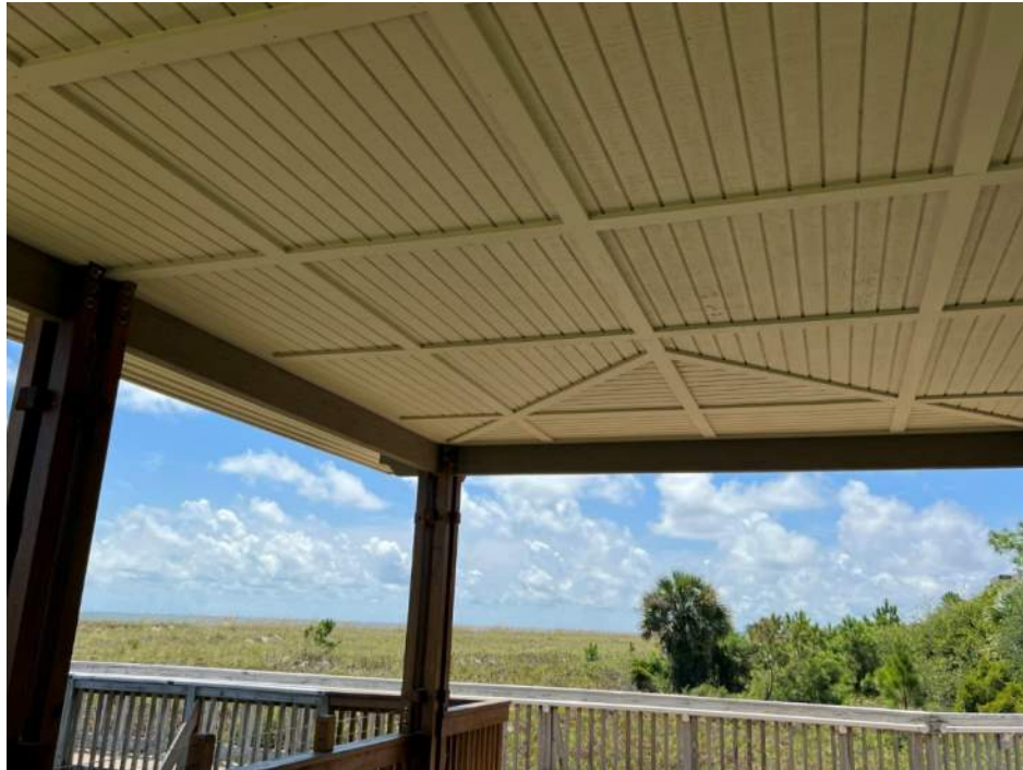
Painted beams and ceiling.
