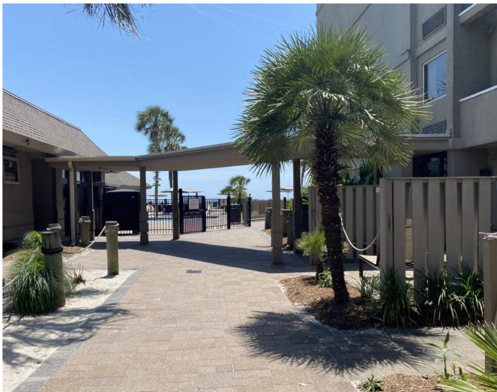
VIEW OF POOL DECK + GATE FROM WALKWAY CORRIDOR
