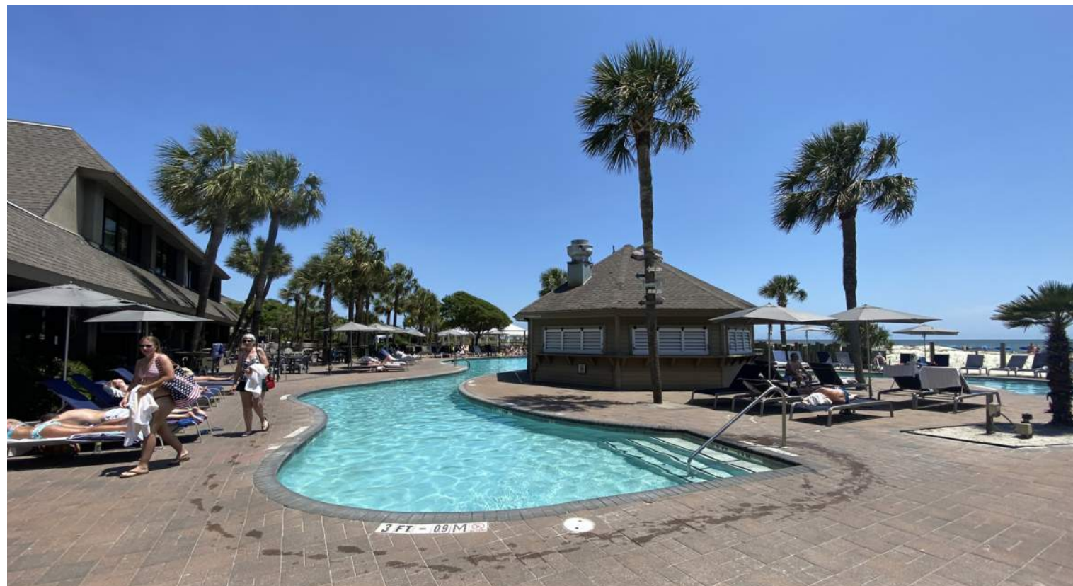
WEST VIEW OF POOL DECK
