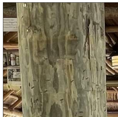
WD-02 WOOD RAILING WOOD MATERIAL/COLOR: MATCH DECKING WD-03 CABLE COLOR: STAINLESS STEEL
