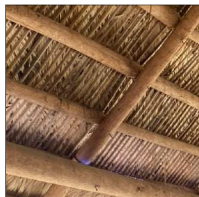
WD-07 NEW WOOD BEAM AND RAFTERS WOOD SPECIE: SOUTHERN YELLOW PINE MATCH EXISTING COLOR: CLEAR COAT NATURAL STAIN & SEALER
