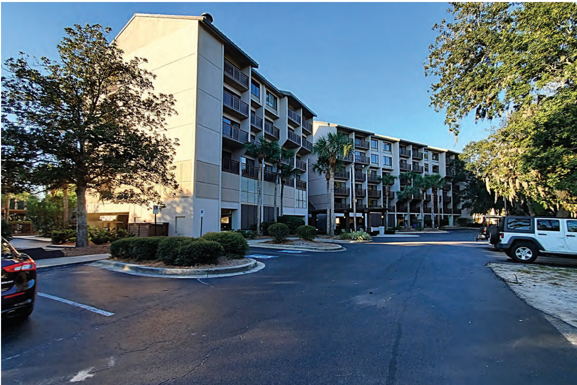
Building View at Northern End looking south
