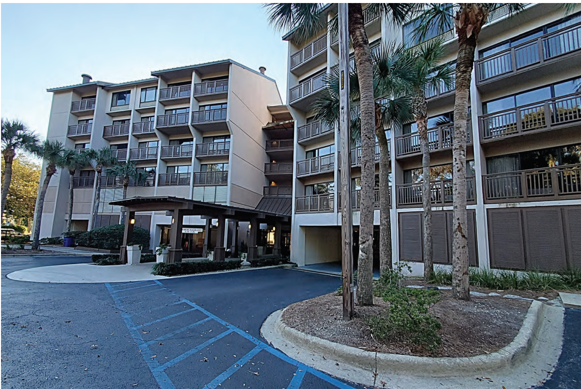
Building Entry looking North
