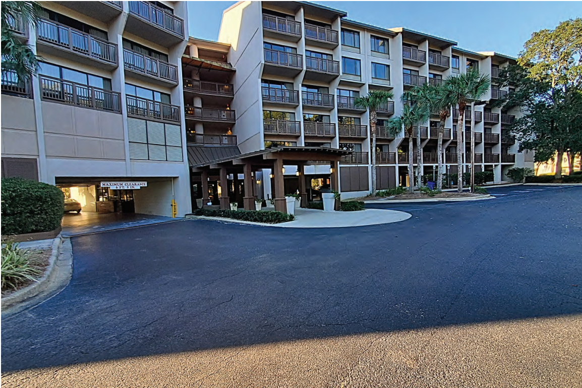
Building View at Existing Entry
