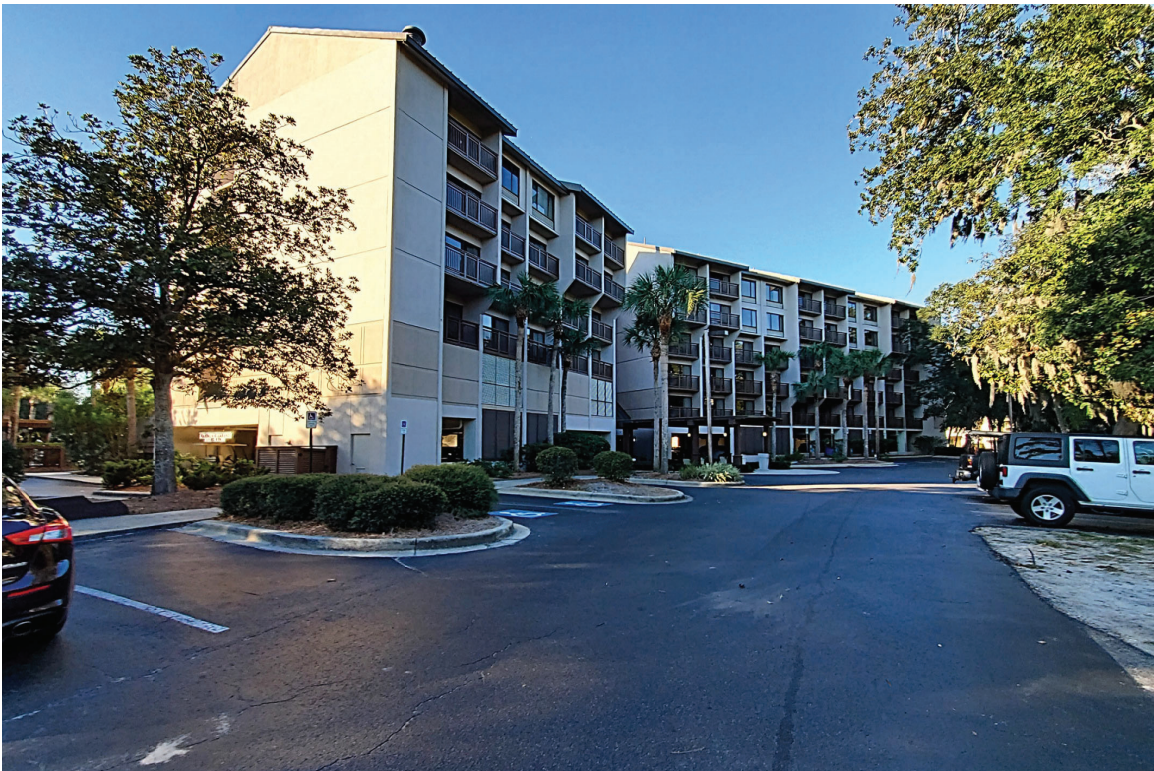
Building View at Northern End looking south
