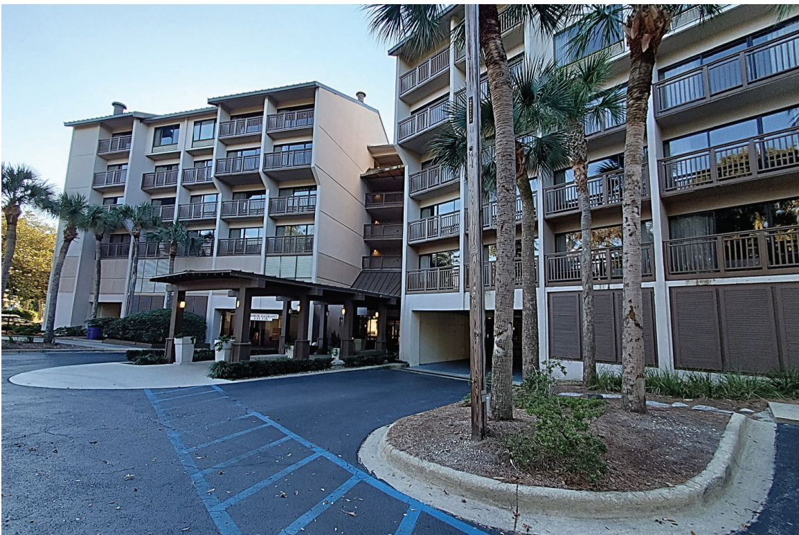
Building Entry looking North
