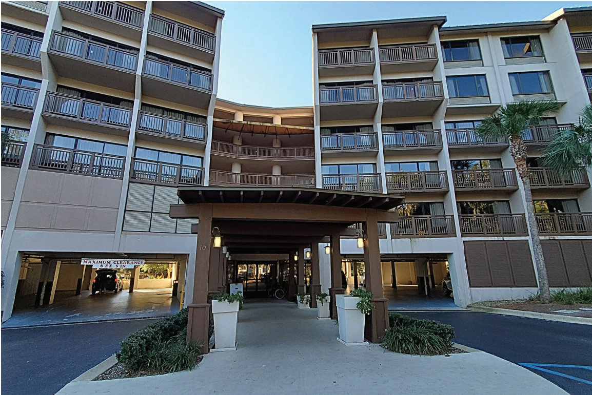
Existing Building Entry
