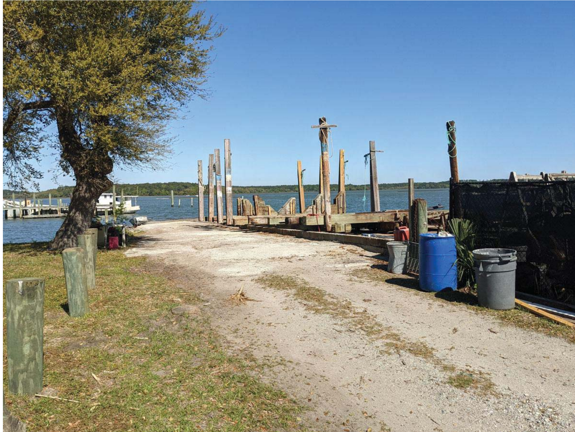
EXISTING RAIL LINE BOAT SERVICE RAMP
