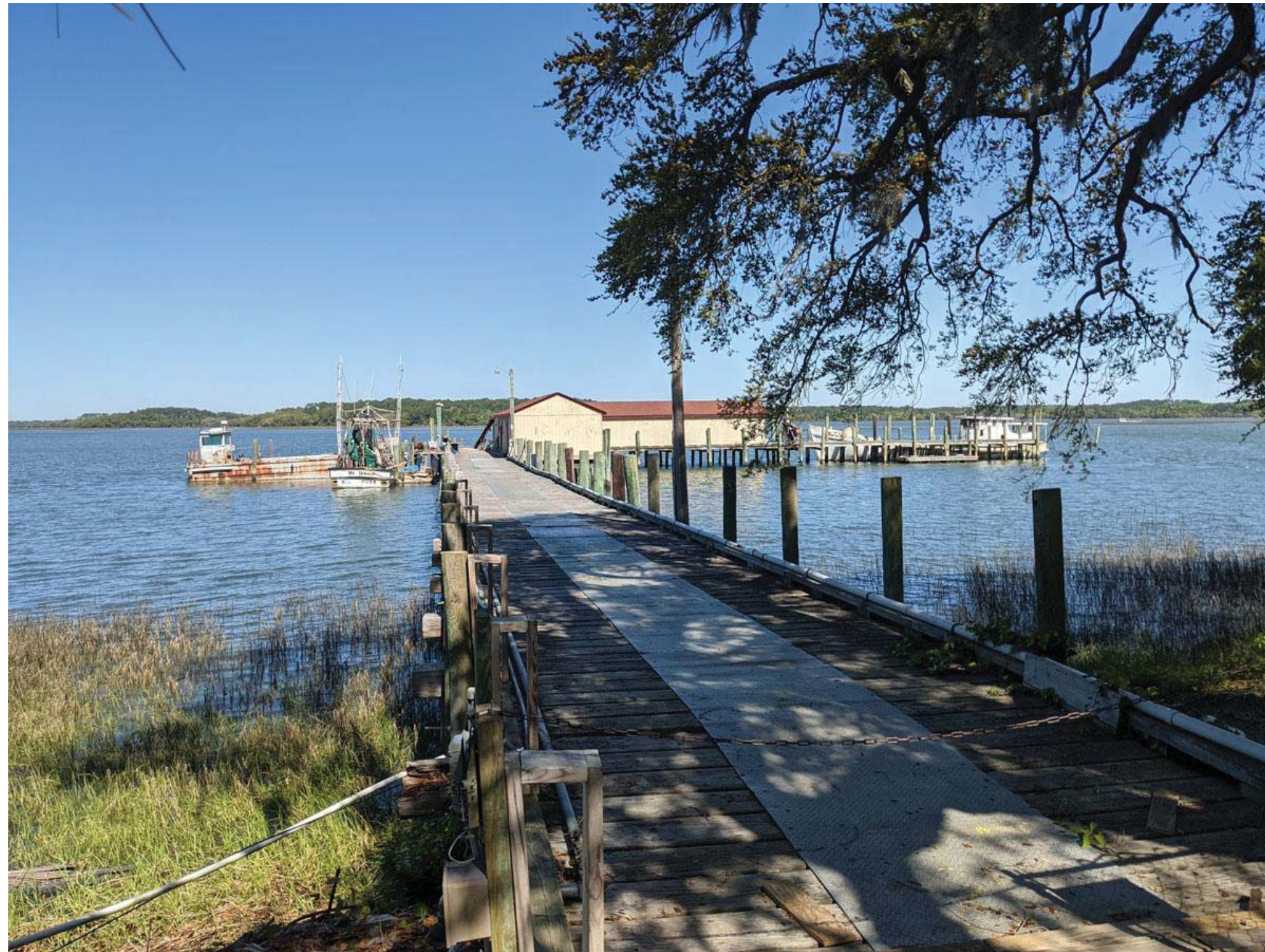
EXISTING DOCK (PROCESSING BUILDING TO BE DEMOLISHED)
