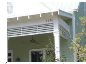
Overhead Louvers (Sim.)
