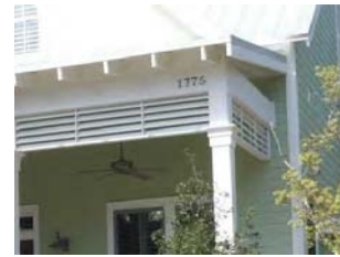
Overhead Louvers (Sim.)
