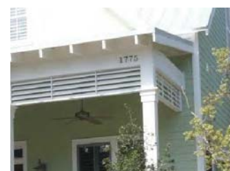
Overhead Louvers (Sim.)
