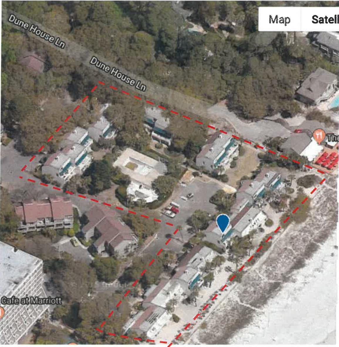
Note brown areas of shingle roof to be replaced are on street side. Areas of green are awnings.
