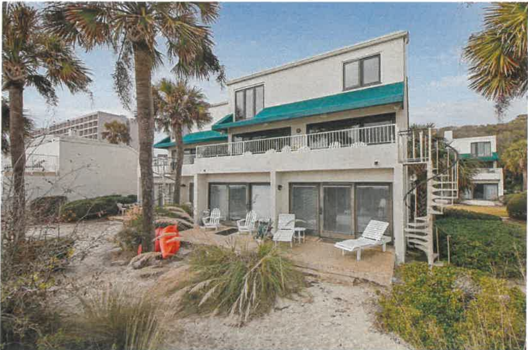
Building 2 (with Bldg. 3 in background)
