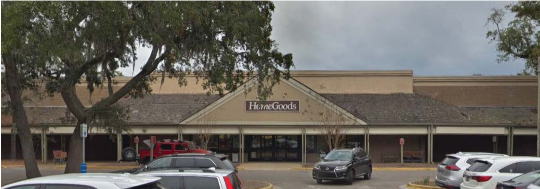
NORTHRIDGE PLAZA HOMEGOODS EXISTING ELEVATION
