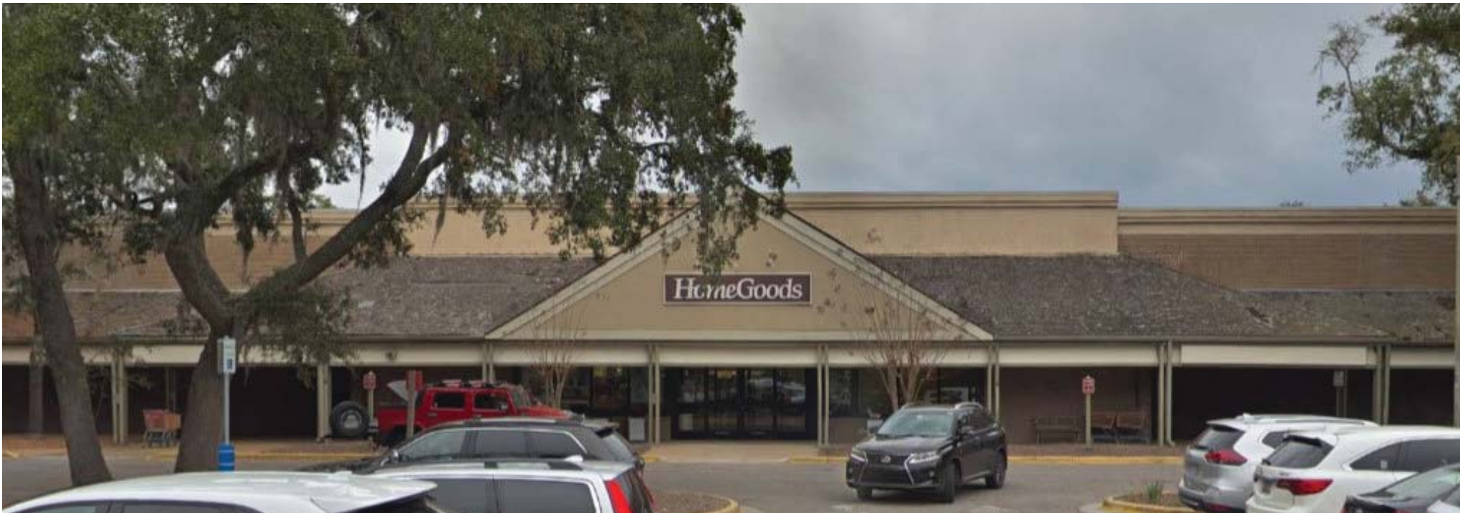
NORTHRIDGE PLAZA HOMEGOODS EXISTING ELEVATION
