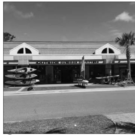
3 FACADE VIEW @ MIDDLE ENTRANCE
