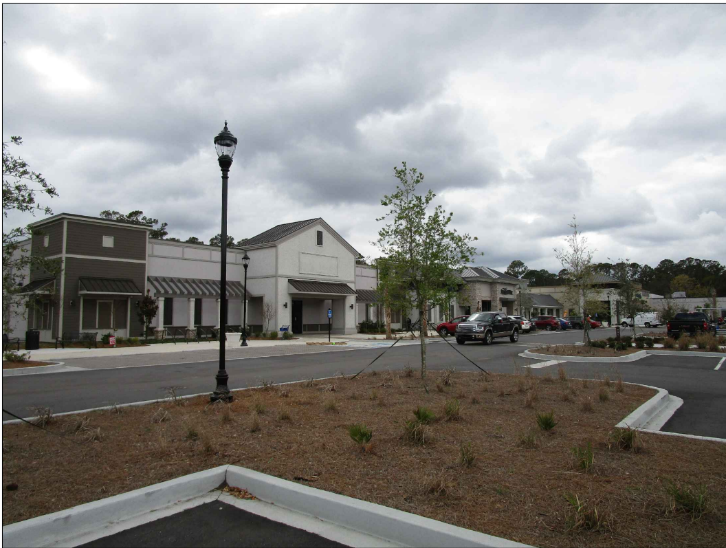
LOOKING WEST AT JR. ANCHORS
