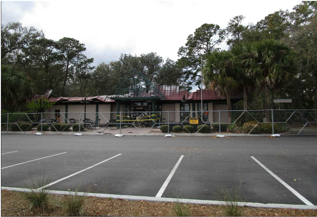
LOOKING WEST AT EXISTING STARBUCKS
