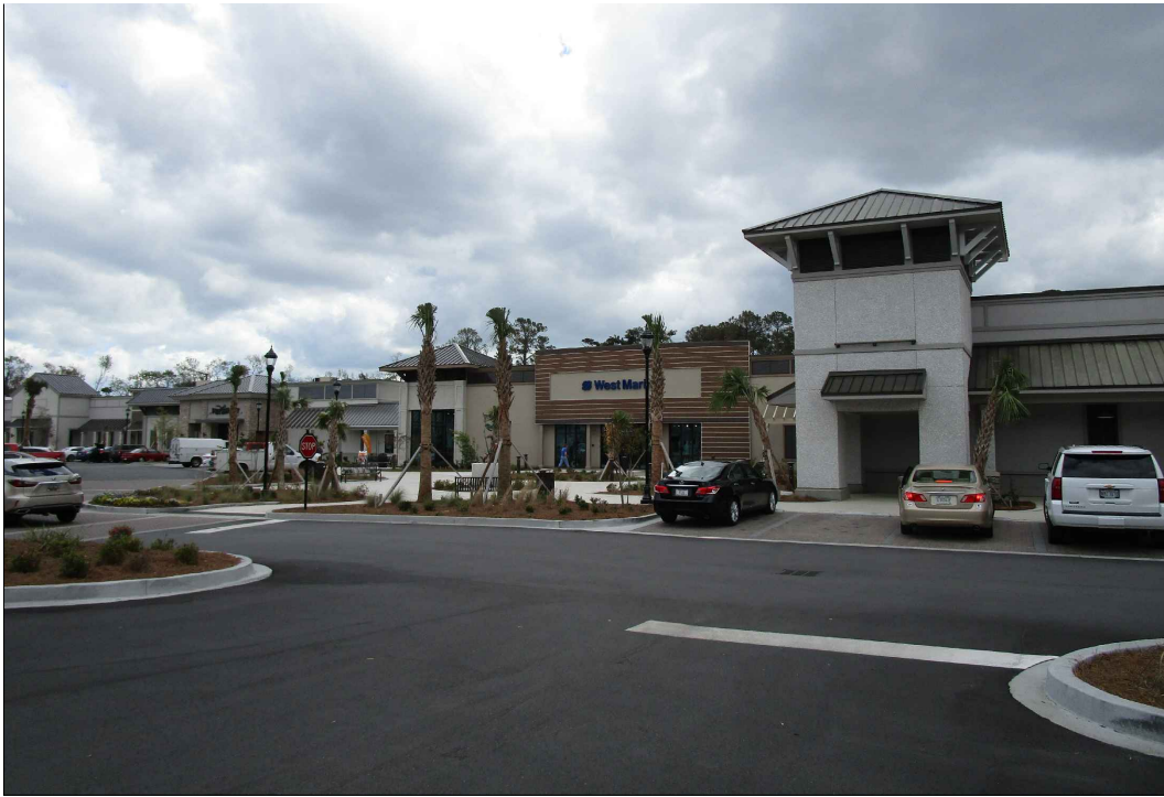
LOOKING SOUTH AT JR. ANCHORS
