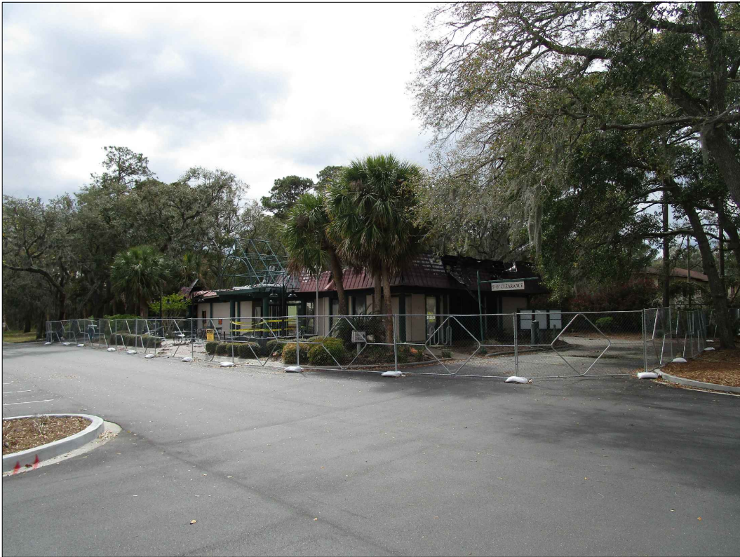
LOOKING SOUTHWEST AT EXISTING STARBUCKS
