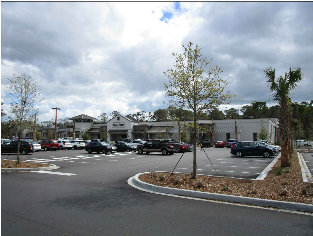
LOOKING SOUTH AT STEIN MART FACADE RENOVATION
