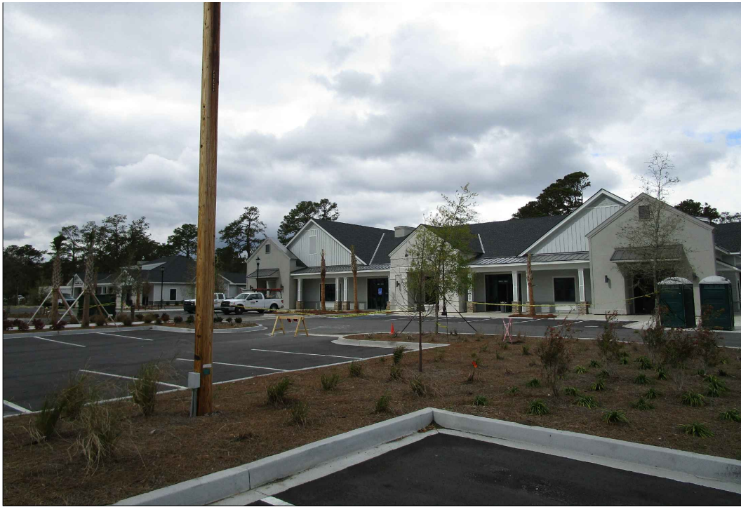
LOOKING NORTH AT BUILDING F
