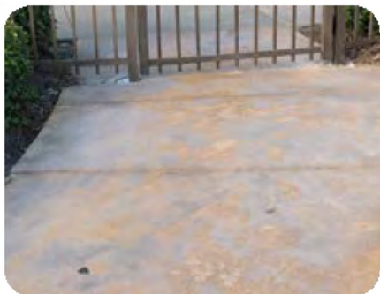
Colored Concrete Walk (Existing)
