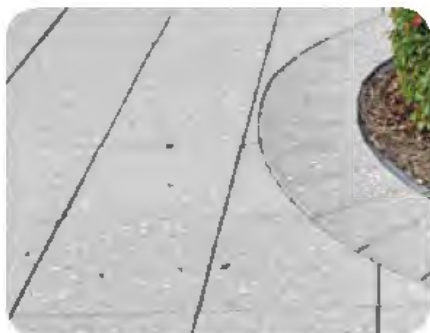
Pool Deck Pavers & Banding (Existing)
