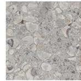
French Porch, Foundation Tabby Stucco Medium Shell
