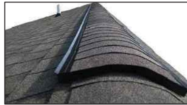
RIDGE VENT FOR SHINGLE ROOFING MANUFACTURER: GAF COBRA 3 FINISH: COVERED WITH ASPHALT SHINGLES
