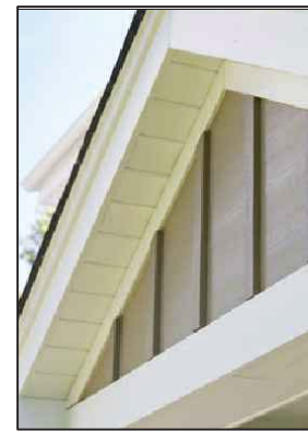
BOARD & BATTEN (SMOOTH) MANUFACTURER: JAMES HARDIE COLOR: SEE RENDERINGS FOR SCHEME
