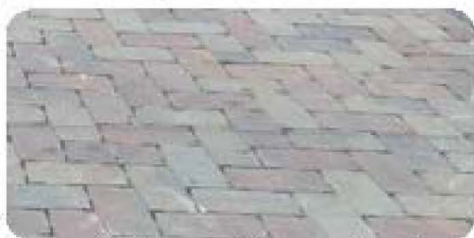
Permeable Pavers - Driveways Type 1
