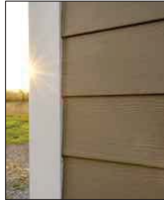
LAP SIDING (SMOOTH) MANUFACTURER: JAMES HARDIE COLOR: SEE RENDERINGS FOR SCHEME
