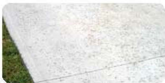
Concrete Walk (Natural - Rocksalt Finish)
