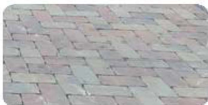
Permeable Pavers - Main Entry (Parking)- Type 1
