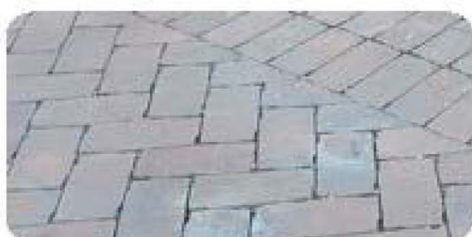
Permeable Pavers - Main Entry (Drive Aisles) - Type 2
