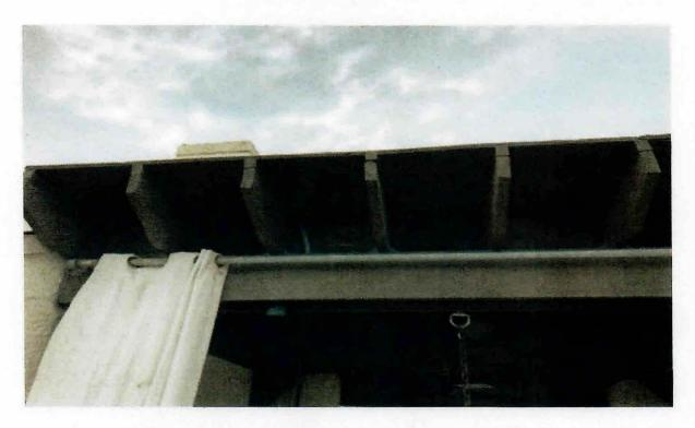
This is the side of the canopy facing Palmetto Bay. Blocks are to be placed between the ceiling rafters, on top of the beam at every space between the rafters and nailed as shown in the previous detail. This is to be done with all ceiling rafters.
