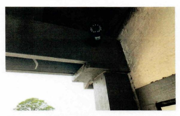
This is typical of the westerly outside post and beam connection. On both ends of this beam, the beam must be tied to the post with 16-gauge coil strapping, that is 12 inches long on each member (post and beam. The post is to be anchored to the wall with HDG %" carriage bolts. A block is to be placed on the sheetrock wall on the inside to span between not less than 2 existing wall studs. 1" HDG washers are to be used on the bolt. Place 3 bolts @ 18" o.c. in the wooden post.
