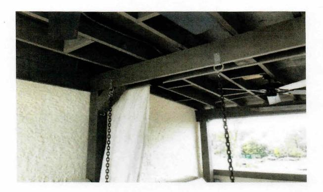
The post to the right in the picture above is closest to the exterior of the deck and it too, needs to be bolted to the concrete block wall with ½" red head bolts with a minimum penetration into the block wall of 5". The red head is to be epoxied into place with Simpson 2-part epoxy or equal. Place 3 bolts @ 18" o.c. in the wood post.
