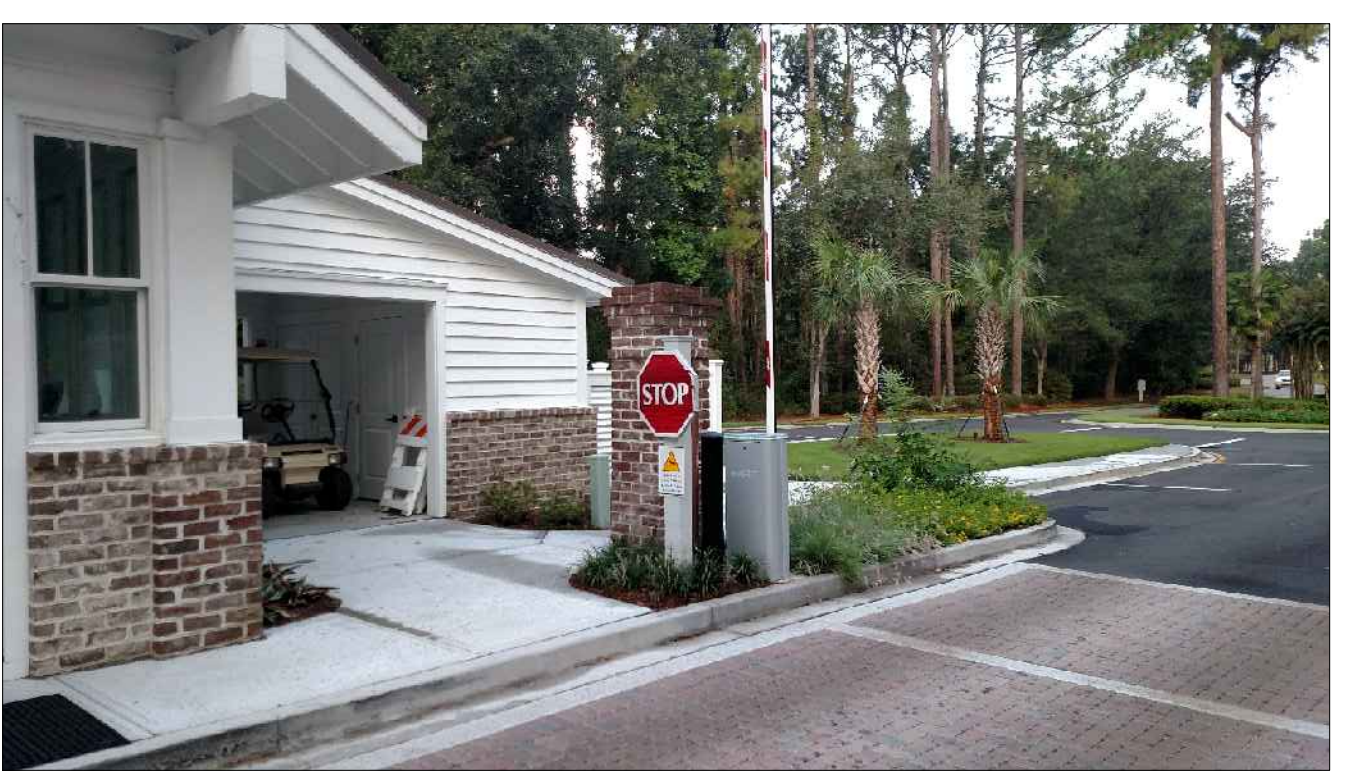
BARRIER GATE EXAMPLE
