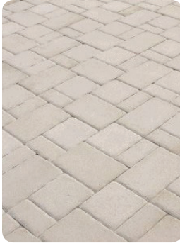
Pedestrian Pavers (Pool Deck)
