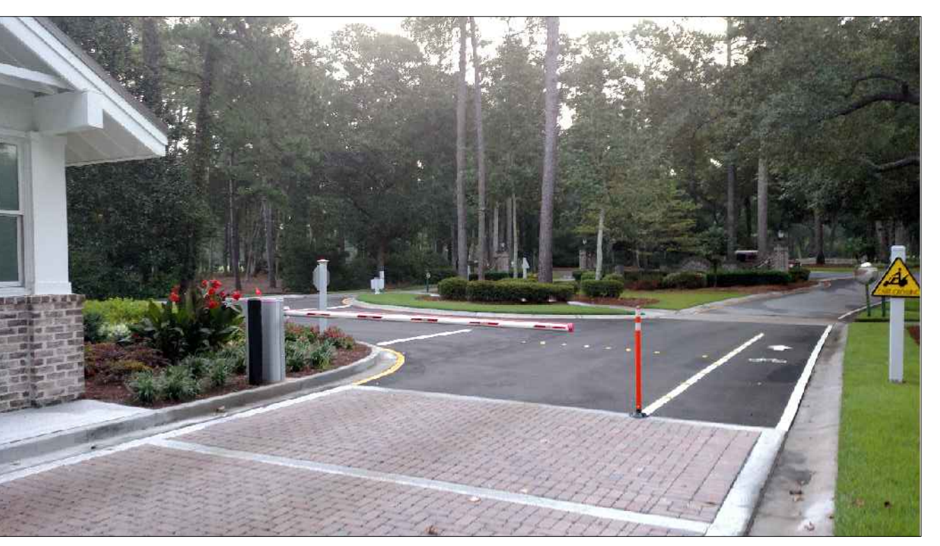
BARRIER GATE EXAMPLE
