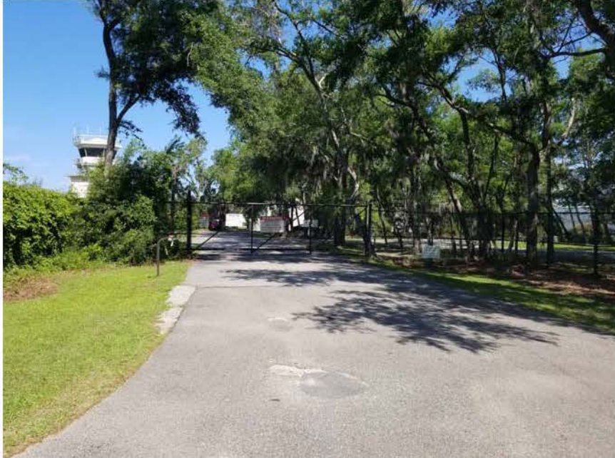
Air Traffic Control Driveway (JKT 06/01/2018)
