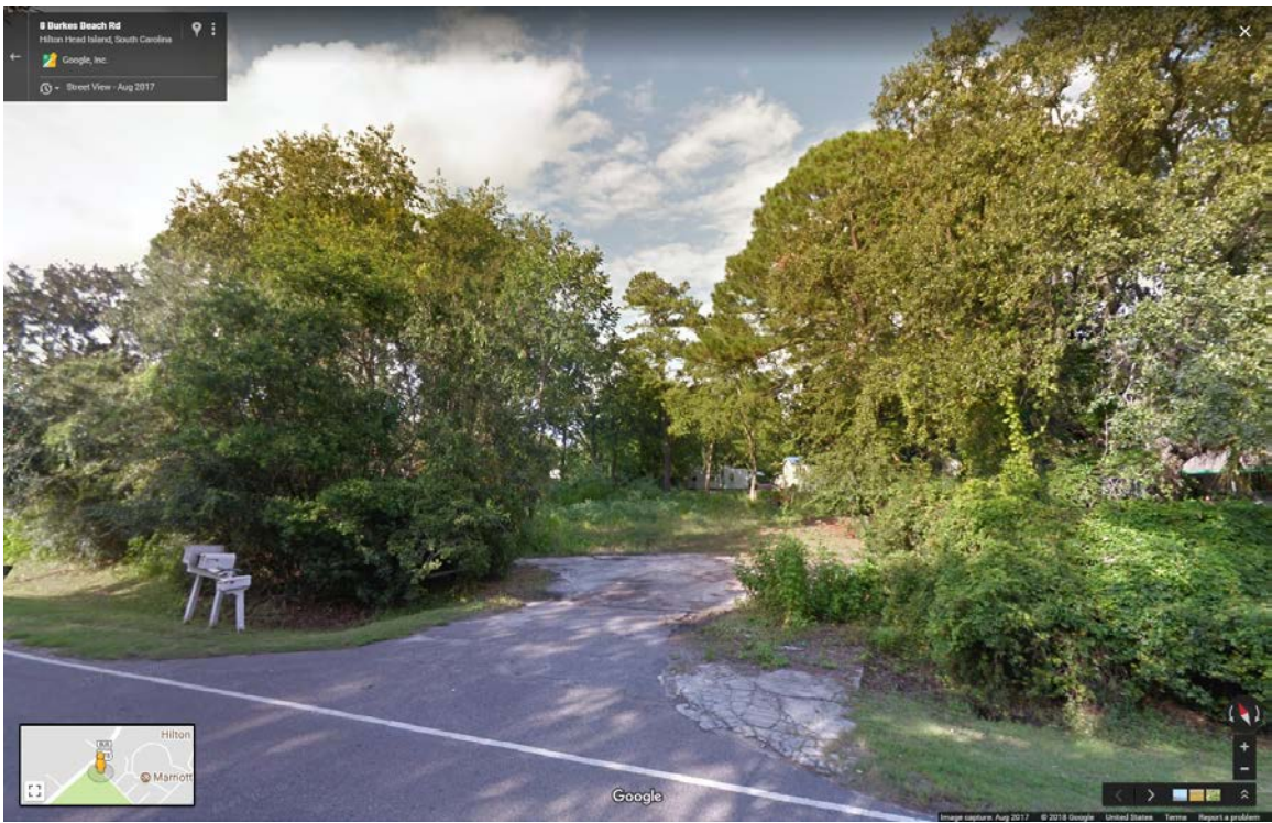
Existing site access at Burke's Beach Rd
