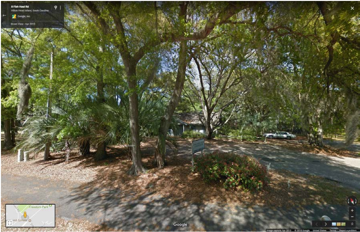
Existing Vet's office on Fish Haul Rd
