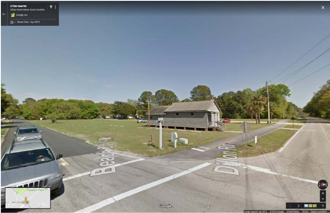
Corner view at Beach City Rd & Dillon Rd
