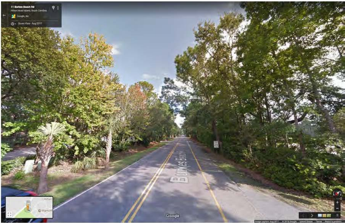
BB Rd looking towards beach direction
